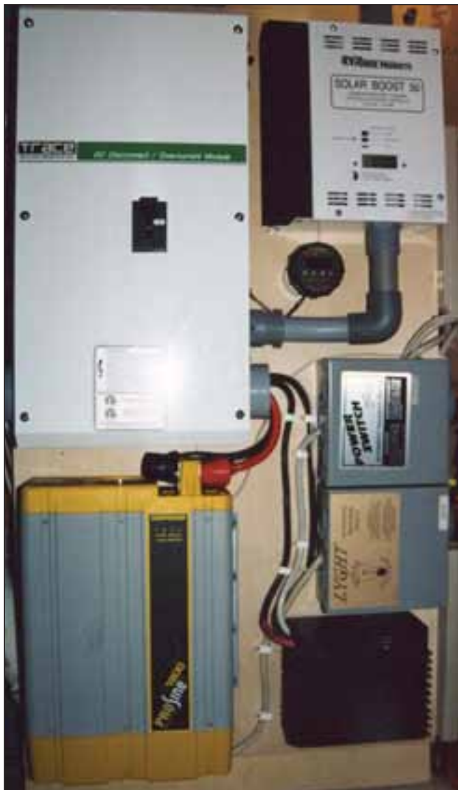
The new power panel with two inverters, charge controller, transfer relays, and overcurrent protection breakers for safety.
