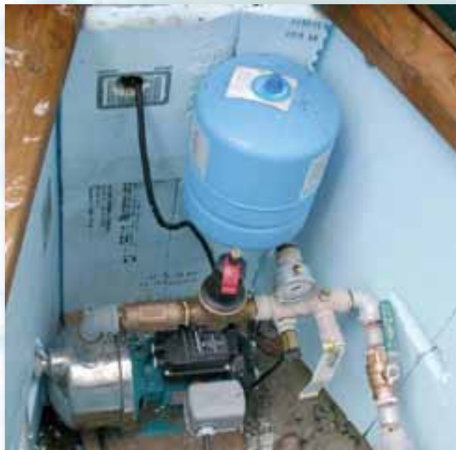
The basic components of a rainwater irrigation system, including pump and pressure tank, in an insulated box.
