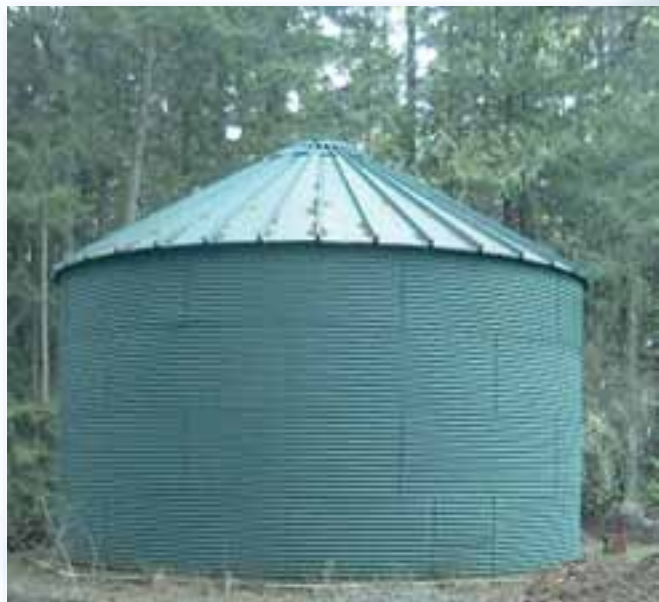
This 27-foot-diameter, 14-foot-tall, steel storage tank, lined with an FDA-approved PVC liner, can store about 58,000 gallons of rainwater.
