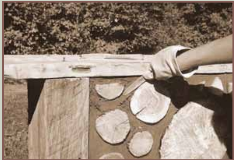
Smoothing and pointing the mortar is the final step.
