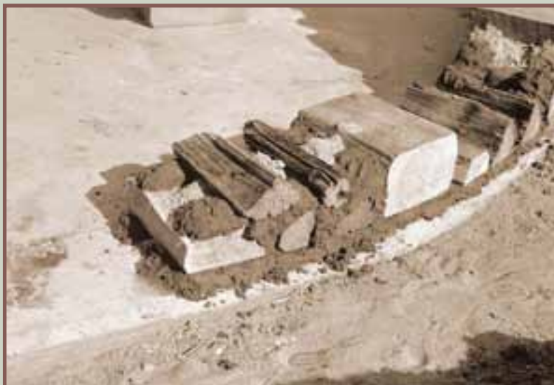
The second course of wood laid on top of the second course of mortar.
